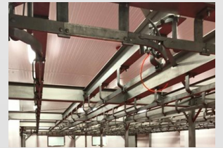
Data Center Structural Supports
